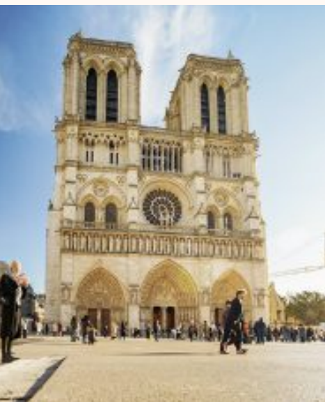
Below: The freshly restored Notre-Dame cathedral
